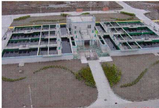
Lamella Plate Settler (Multiflo / Actiflo)
