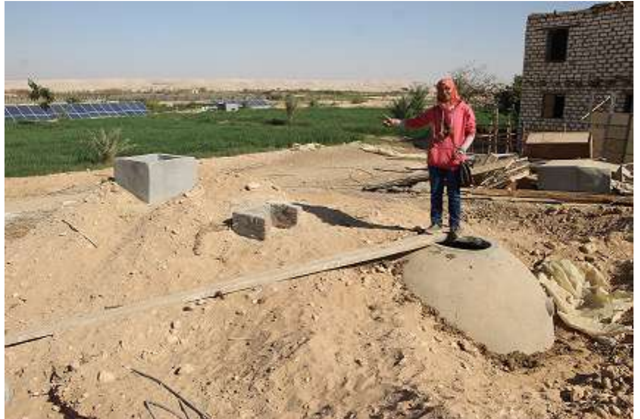
PV pumping and biogas at a rural farm in Altoud - Luxor
