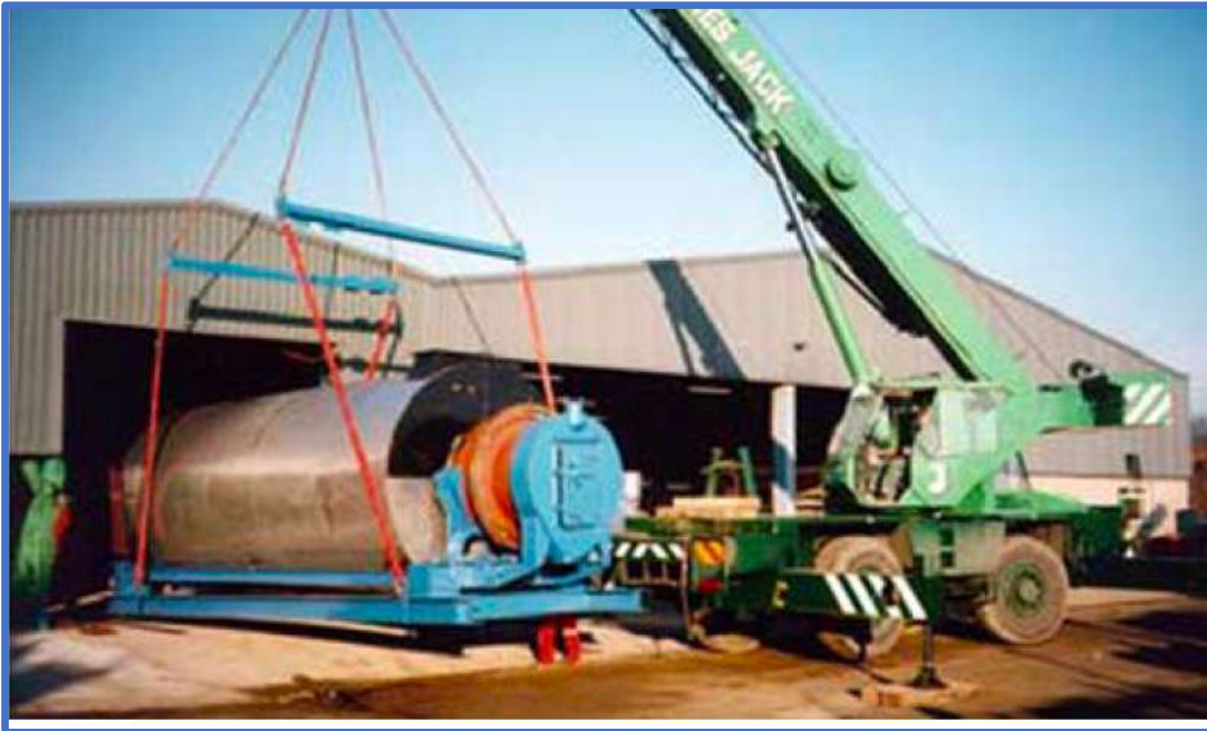
Delivery of a rotary dryer
