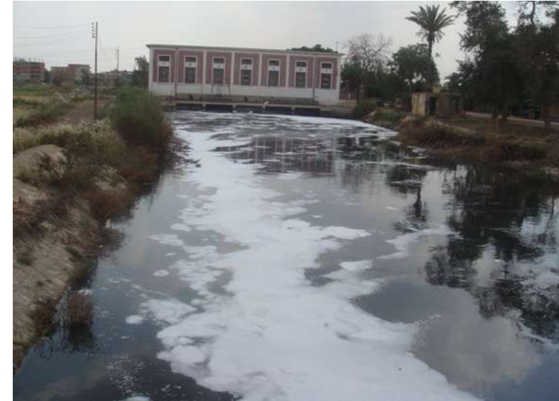
Mixing station feeding Khadrawiya drain to Al Abbassa main canal
