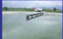
Sludge Lagoon System Completed : 1 Nos
