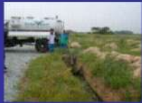
Trenching System Completed : 25 Nos
