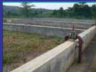
Drying Beds Completed : 3 Nos
