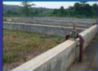
Drying Beds Completed : 3 Nos
