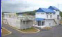
Dedicated Centralised Sludge Treatment Completed : 8 Nos
