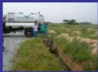
Trenching System Completed : 25 Nos
