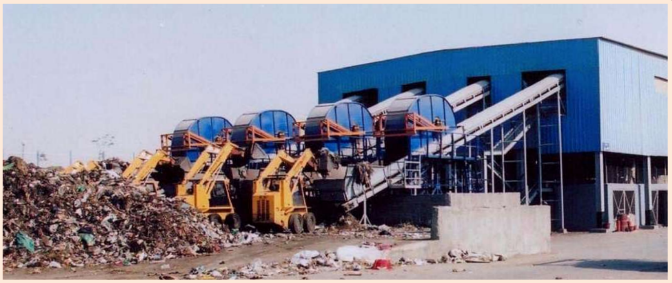
Reception area and feeding system in 15 th of May Facility
