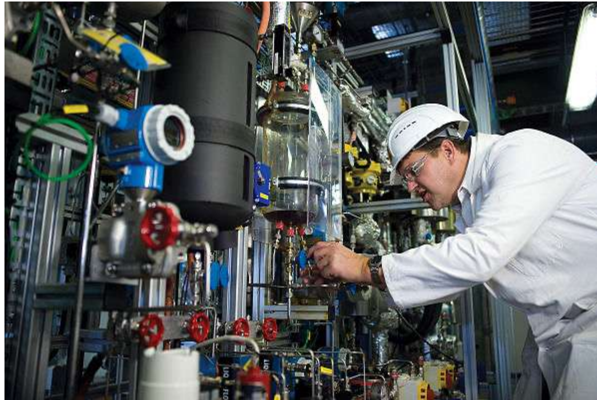
Figure 8 The pilot plant for the new OMEGA process to make ethane-1,2-diol.
