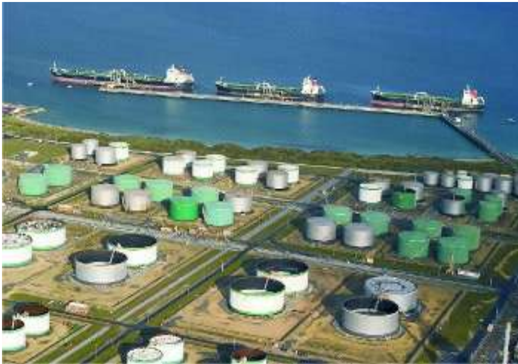
Figure 4 Storage tanks and docks at the Kwinana refinery near Perth, Western Australia.
